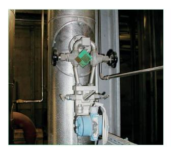
There are many procedures available for measuring the flow of water. Yet even with this medium there are certain application areas in which SDF sensors are the only reasonable choice.
